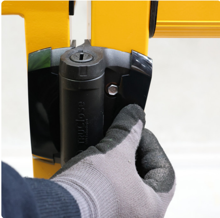
▲ Screw the top hinge first to the post
