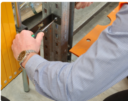
▲ Position bottom wall bracket and secure
