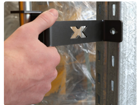
▲ Position top wall bracket and secure
