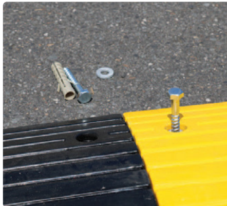
▲ Reposition hump and insert coach screws
