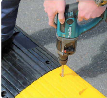
▲ Pilot drill mounting holes
