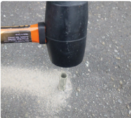
▲ Insert nylon plugs flush with road surface
