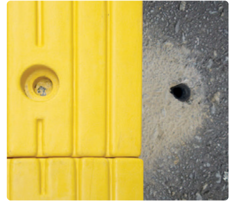
▲ Drill out pilot holes
